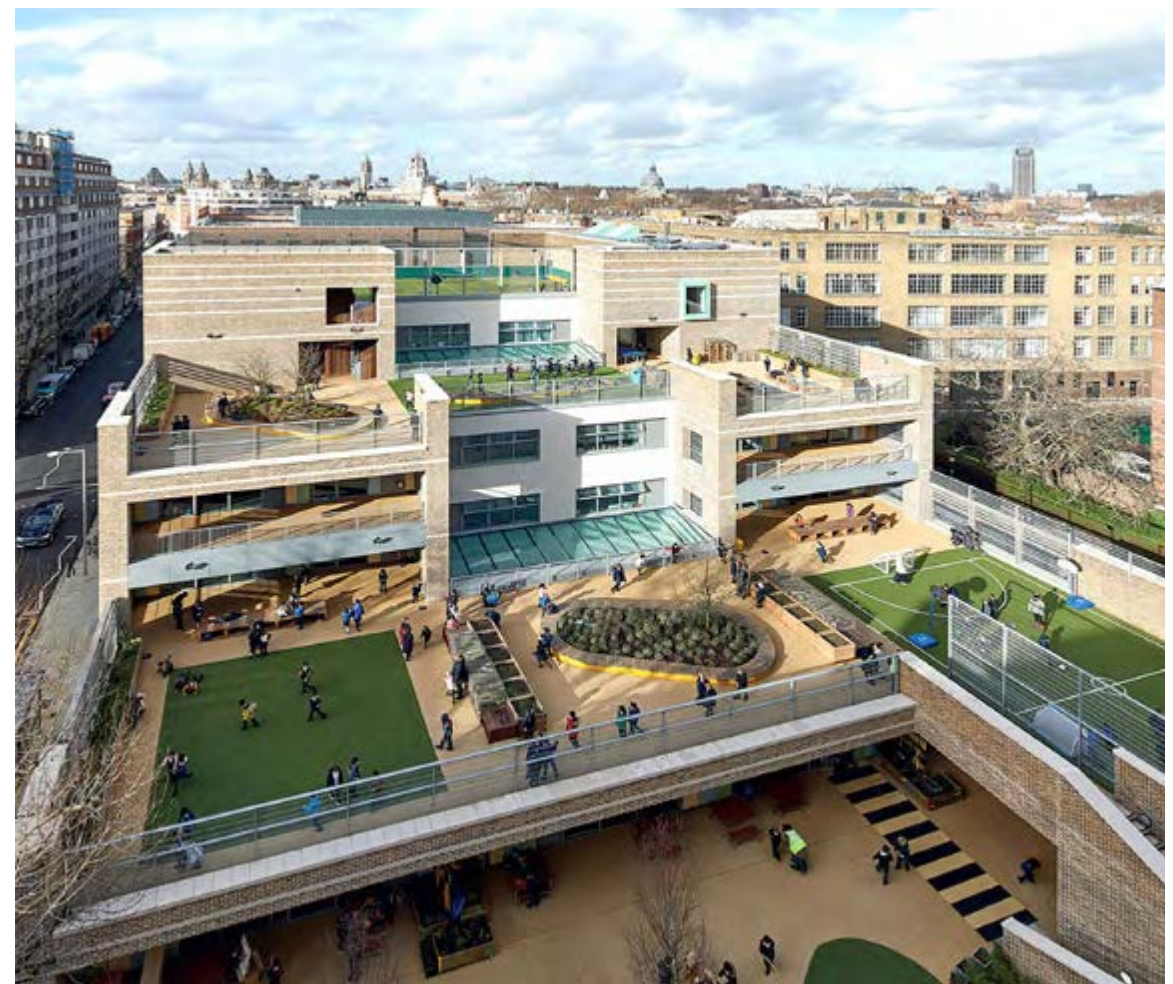
Marlborough Primary School, London, UK, Dixon Jones, fot. Paul Riddle
