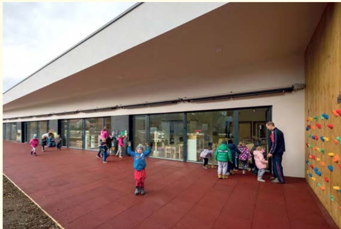
Timeshare School and Kindergarten Podgorje, Jure Kotnik Architect, Podgorje pri Slovenj Gradcu, Slovenia, fot. Janez Marolt
