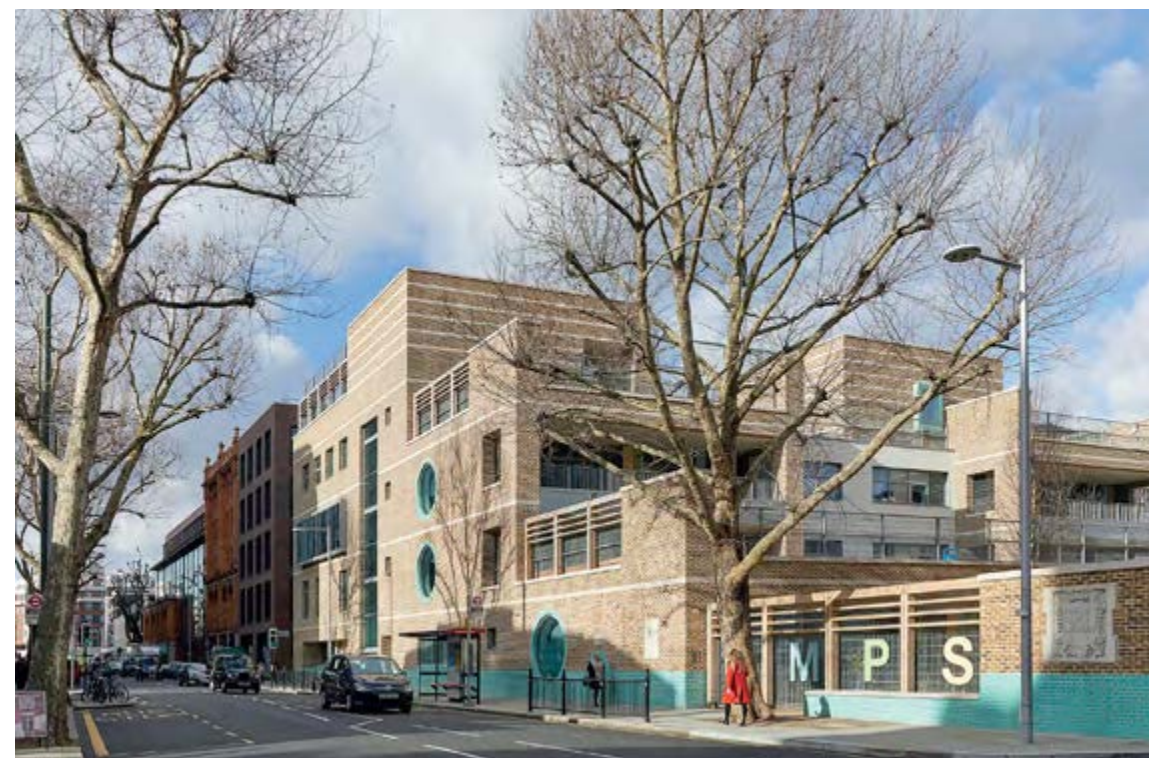
Marlborough Primary School, London, UK, Dixon Jones, fot. Paul Riddle
